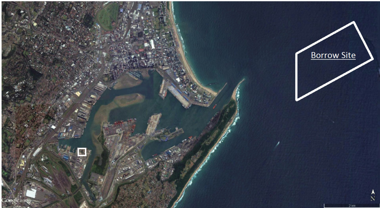
Figure 1.3-1: Satellite Image Showing the Location of the Offshore Borrow Site and the Lot 10 Casting Yard.
